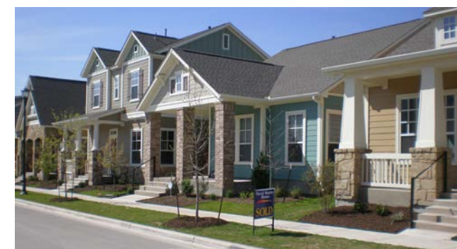
Mid-density residential can take a variety of forms, including townhomes, three or four plexes, or small multifamily developments (image source: City of Austin).
